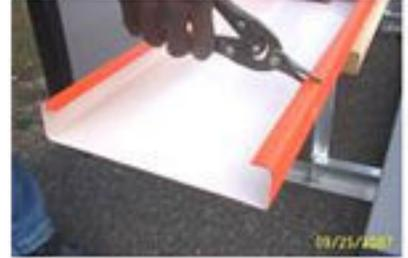
If you need to notch the bleachers covers, start by aligning a piece of Perma-Cap in position. Use a felt tip marker to draw the cutting marks on the underside lip of the vinyl. Make the cut marks about 1/2 inch out from either side of the brace. Use ordinary tin snips to cut the vinyl along the lines.
