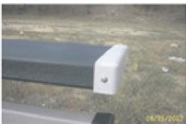
Slide the end caps over the end of the bleacher and secure with a screw, front and rear as shown.
