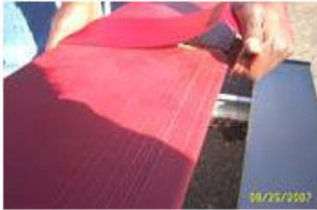
Pull the other end of the Joint Cover over the front edge of the cap until the lower lip snaps underneath the bleacher.
