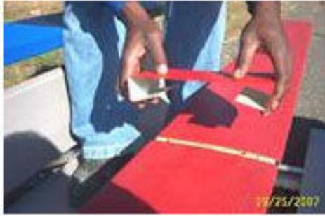
When installing Perma-Cap covers end to end, leave at least a 1" gap. Use a Joint Cover to finish the cap.
