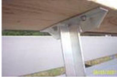
The Perma-Cap cover should snap easily over seat. On some bleachers, the support brace underneath may be mounted close to the front or rear edge of the seat. Do not try to fit the cover over the brace, the vinyl must be notched to fit.
