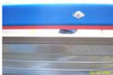
The spacer will help you gauge how far to drive the screw.
