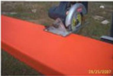
If needed, Perma-Cap bleacher covers can be cut to shorter lengths using tin snips, shears, or a circular saw with a fine tooth plywood blade.
