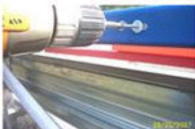
Do not screw the cover tight against the board. They must be able to move freely allowing the cover to expand and contract with temperature changes.
