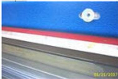
Push the Perma-Cap cover toward the playing field, so it is flush against the back of the bleacher. Snap a plastic spacer into the center of the screw slot. Drive a screw through the spacer.
