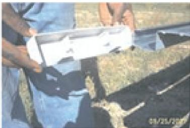
The end caps are manufactured with 4 taps on the inside of the cap. These are used for aligning the cap onto the Perma-Plank steel.
