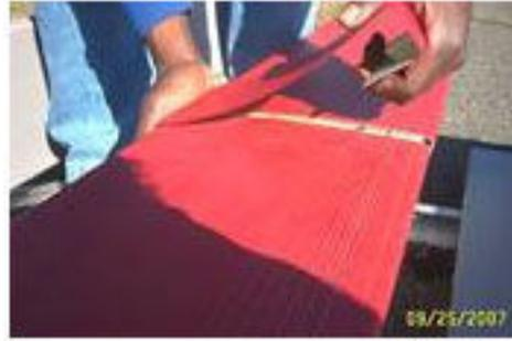
Start with one end of the seam cover and hook the lower lip under the Perma-Cap at the back of the bleacher.
