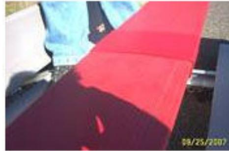
Secure the seam cover to the wood plank by driving a single screw through the holes in the Joint Cover.
