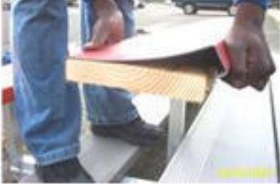
Snap a length of Perma-Cap vinyl onto the bleacher, with the screw slots toward the back. First, hook the front edge of the vinyl cover over the bleachers and starting at one end, stretch the cover over the back of the board. Push down on the back of the cover until it snaps into place. Continue this process over the length of the cover.
