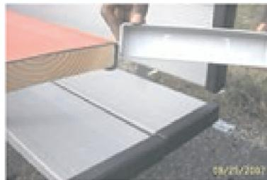
When covering either wood or aluminum planks, these taps must be removed.
