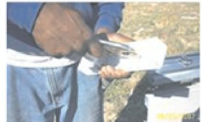
This is easily done by simply using a pair of pliers by prying back and fourth until they snap off.
